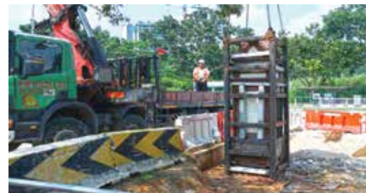
The pillars were chain-lifted by crane onto the back of a lorry (top & below)
